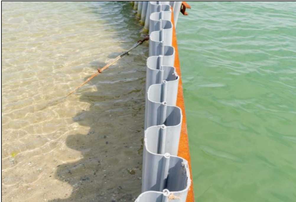
Figure 3-18: A Typical Cofferdam (Source: EIA Report)
