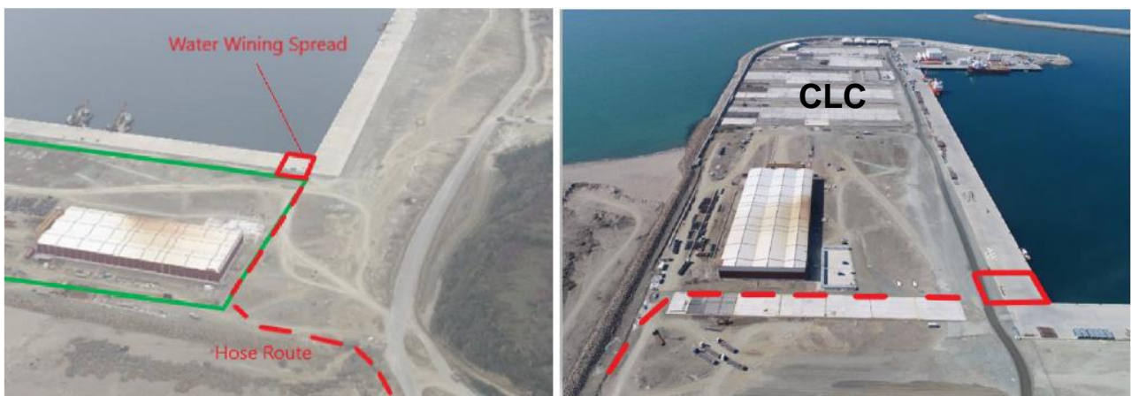
Figure 3-3: Aerial View of Water Winning Spread at CLC
