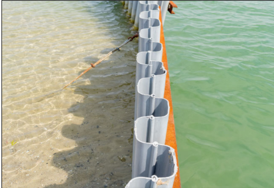
Figure 3-18: A Typical Cofferdam (Source: EIA Report)
